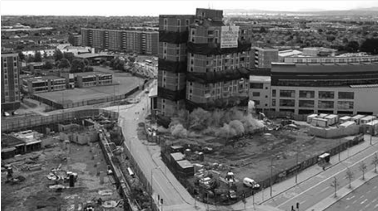
McDonagh Tower, during a controlled implosion bringing the block down as part of the Ballymun Regeneration project in 2005
